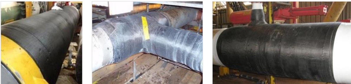
Photographs courtesy of TEAM Inc.
