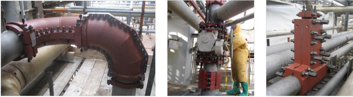
Photographs courtesy of TEAM Inc.
