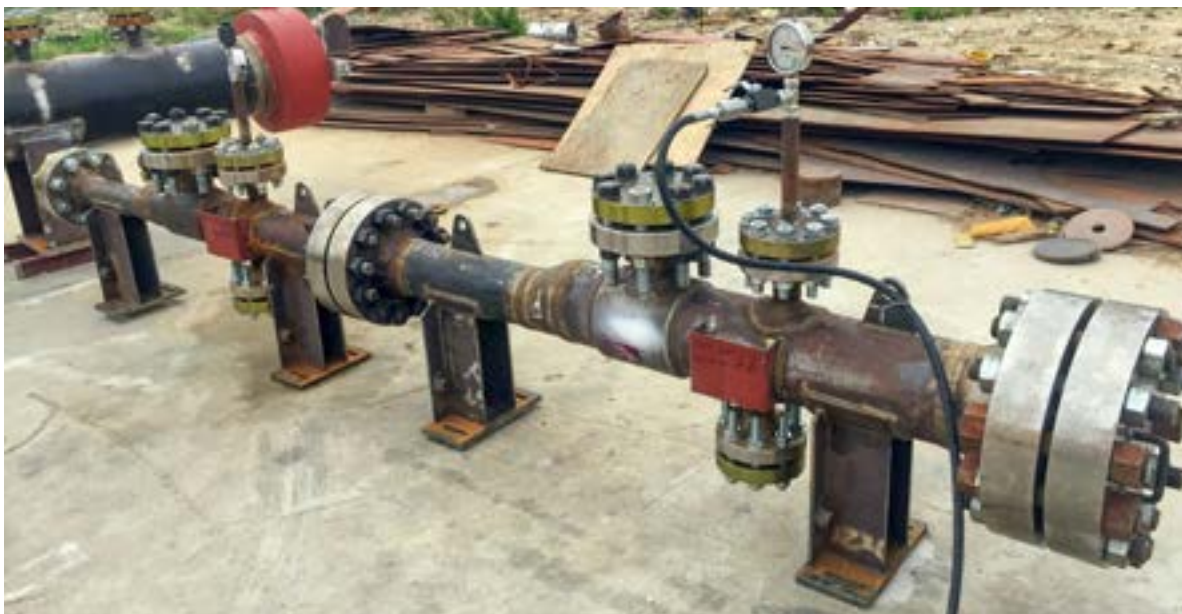
Example layout of a high pressure piping spool being pressure tested
